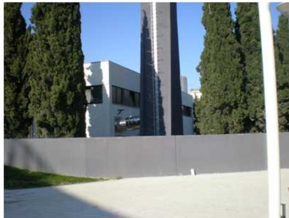
KBC SPLIT – FIRULE, (instalirana snaga 12,5 MW)
